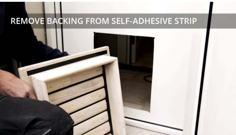
GLUE DOOR WITH SELF-ADHESIVE STRIP
