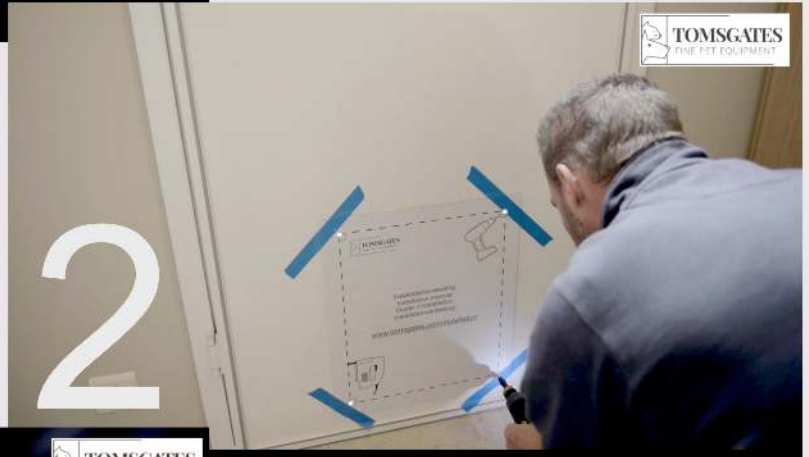
Drill holes in the corners
