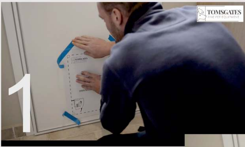
Apply the installation template
